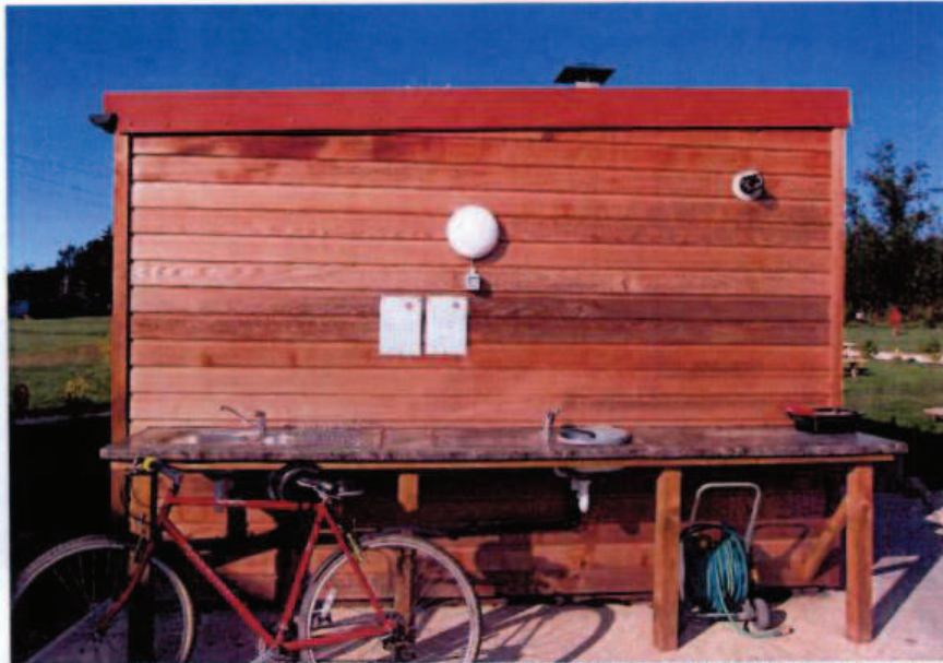
Photograph 3 the south west elevation showing the 2 sinks available for the use of camping visitors
