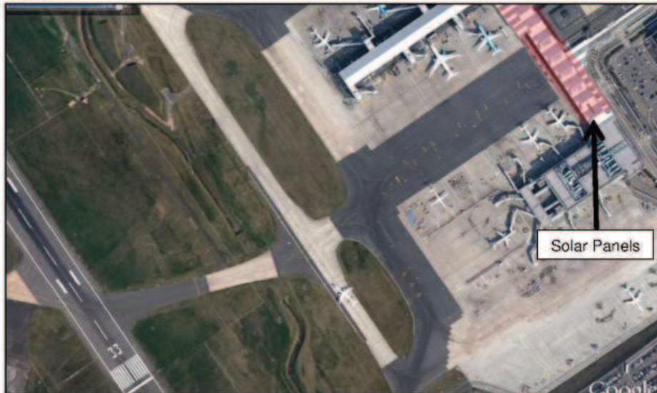
Figure 19 Solar panels at Birmingham Airport
