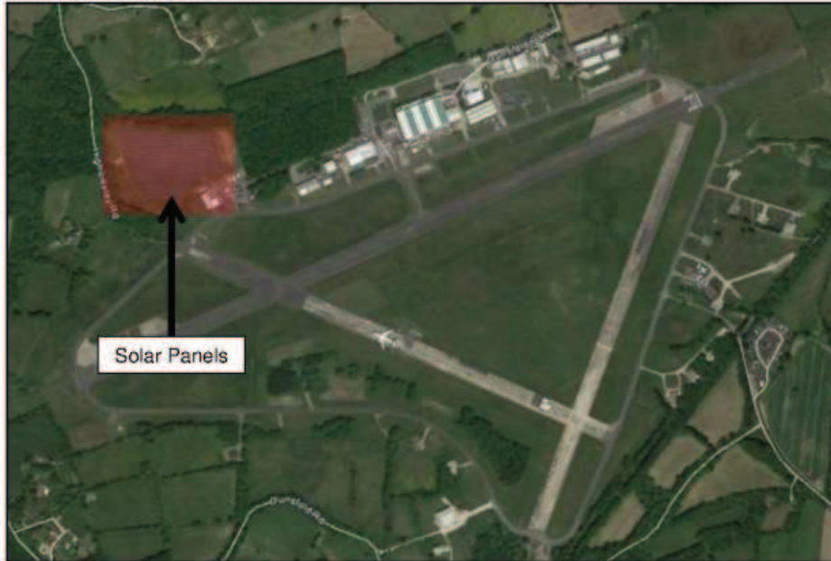
Figure 18 Solar panels near Dunsfold Aerodrome
