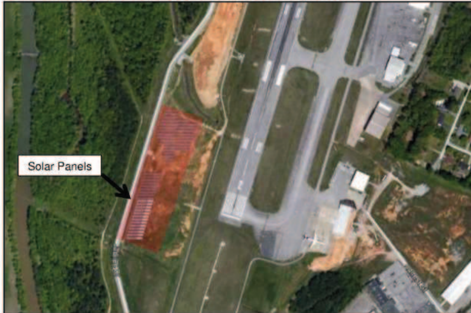
Figure 20 Solar panels at Chattanooga Airport
