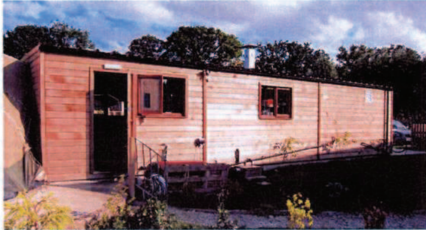
Photograph 1 The Camp Kitchen from the north west
