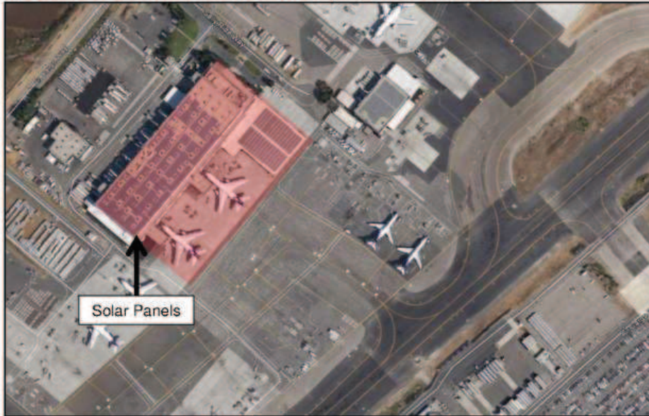
Figure 24 Solar panels at Oakland International Airport
