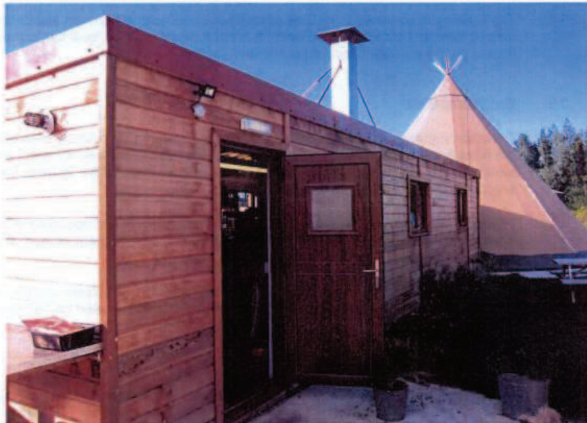
Photograph 2 The Camp Kitchen from the south showing its relationship to the Canteen Tent or Café
